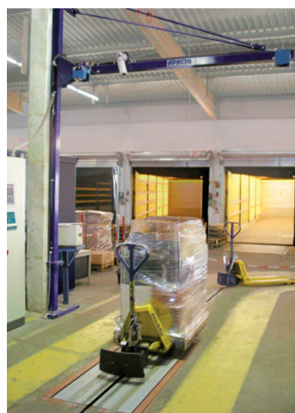
Underfloor chain conveyor
